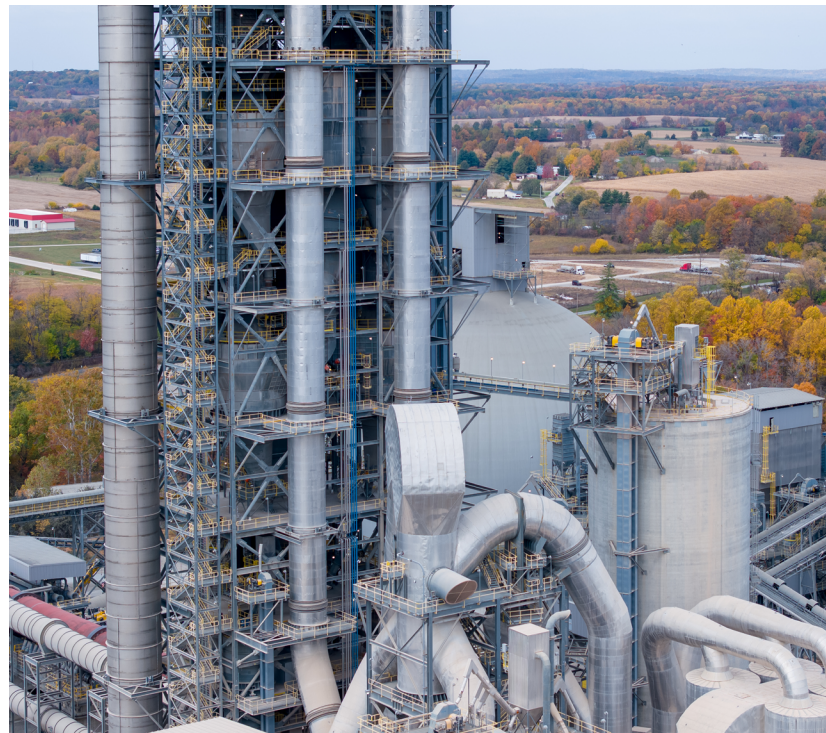
Heidelberg Materials Mitchell Plant – New Cement Preheater-Precalciner Tower.
