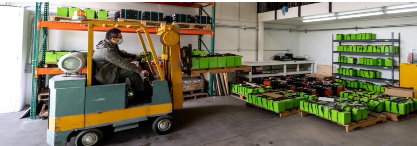
Batteries that once powered electric delivery trucks being prepared for a 2LBESS
