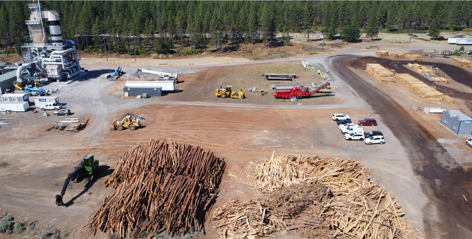
Hat Creek facility view of the feedstock yard
