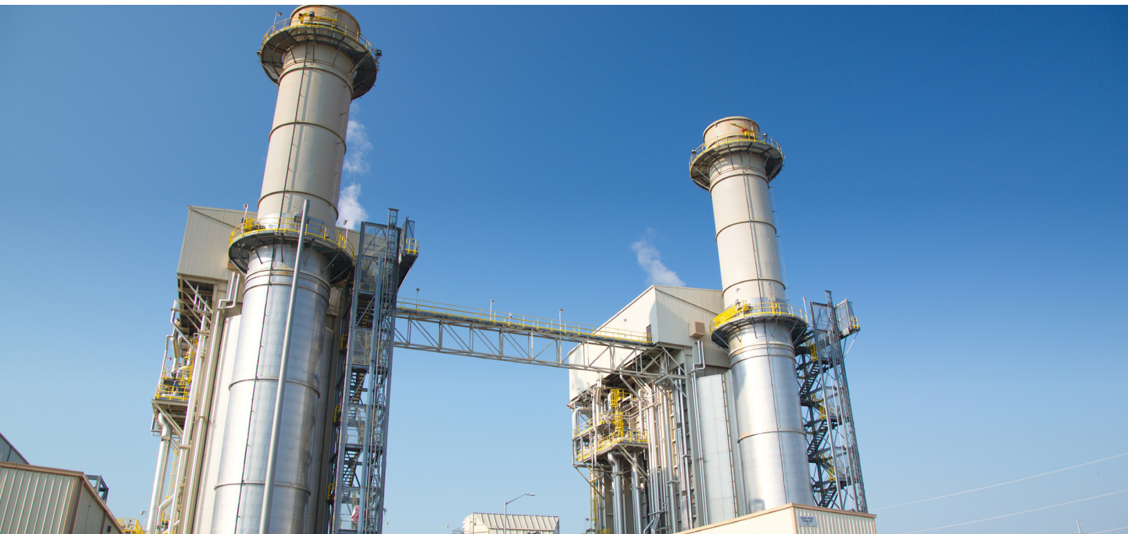
Cane Run Natural Gas Combined Cycle Generating Station in Louisville, KY
