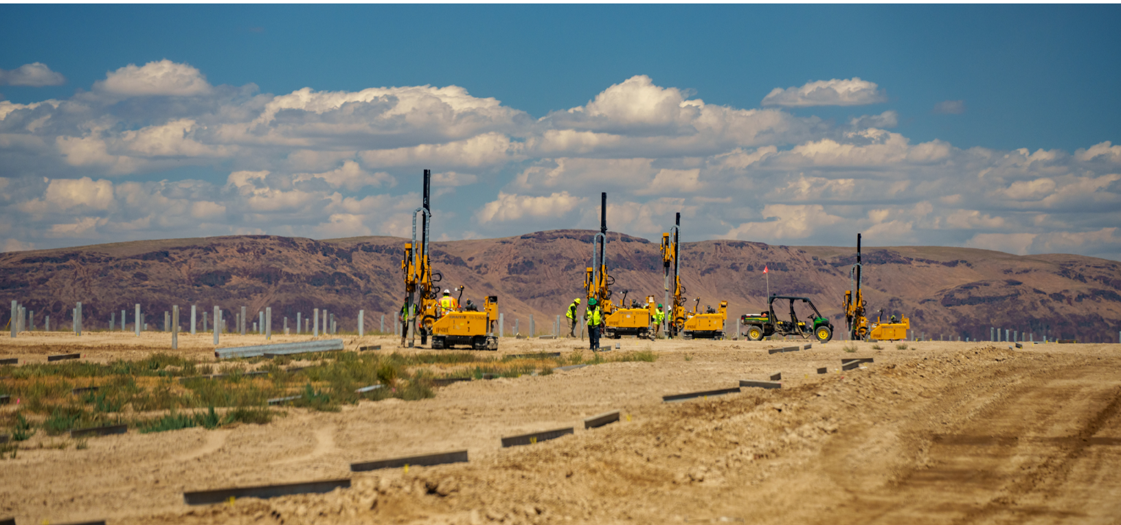
Pile foundation construction in preparation for mechanical installation at Nevada Gold Mines' existing solar facility
